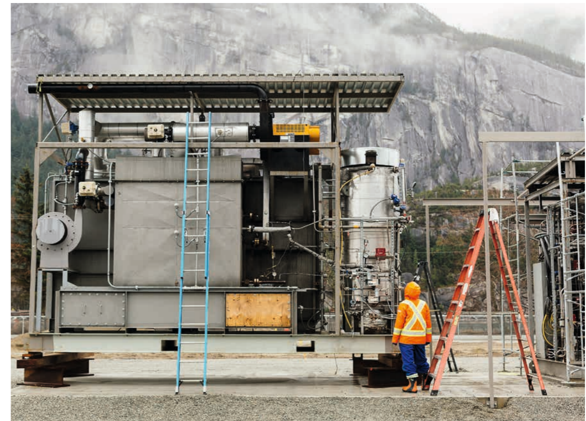
8.10 > This facility captures carbon dioxide from the ambient air and produces fuel from it. It was developed by the Canadian company Carbon Engineering, which is also involved in building the first large DAC plant in the USA.
