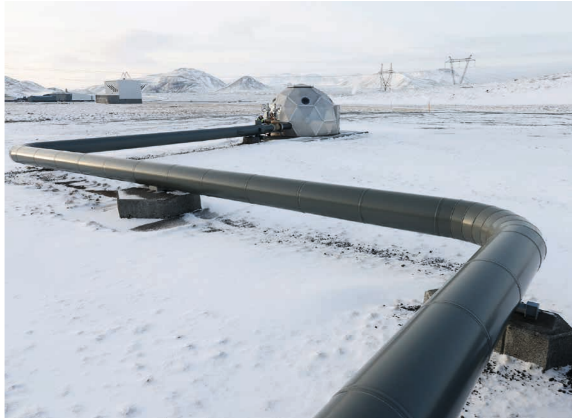
8.20 > This pipeline is part of the CarbFix Project in Iceland. Since 2014, captured carbon dioxide dissolved in water has been injected into the upper ocean crust there.
