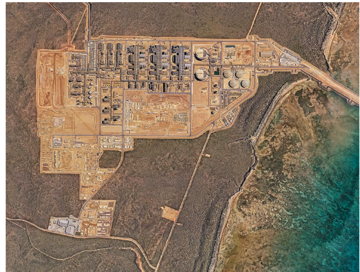
8.13 > At this liquefied natural gas plant on Barrow Island, Australia, carbon dioxide is captured during natural gas processing and injected underground some distance away at a depth of two kilometres.
