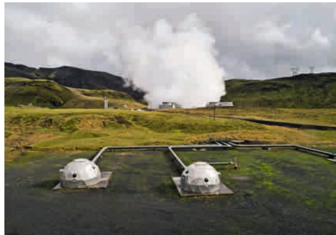
1.26 > Iceland has achieved some small-scale success in removing carbon dioxide from the atmosphere and sequestering it underground. The process involves dissolving the extracted gas in fresh water and injecting it into the warm volcanic basalt rocks. The components of the rocks react chemically with the carbon dioxide, resulting in its mineralization and conversion to rock material itself.
