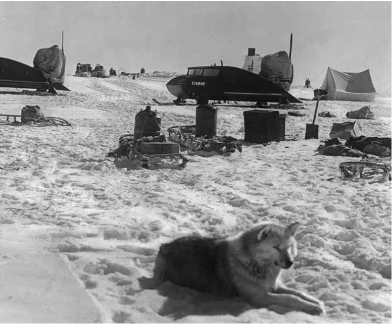
1.29 > A propeller sledge built by the Finnish State Aircraft Factory. The German polar researcher Alfred Wegener had two of these built for his Greenland expedition, but the two vehicles Schneespätz (Snow Sparrow) and Eisbär (Polar Bear) failed to operate properly during the mission.
